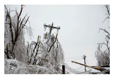
**An avalanche of failure.** Large-scale blackouts can be triggered by small events, such as the failure of a power line like this one in Missouri in 2007, caused by an ice storm. A new model suggests that the explanation for the probabilities of various blackout sizes lies not in the internal dynamics of blackout events but in the distribution of city sizes.
