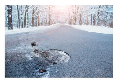
Damage to roads from ice comes from the growth of ice crystals, not from the expansion of water as it freezes—as is commonly thought.
