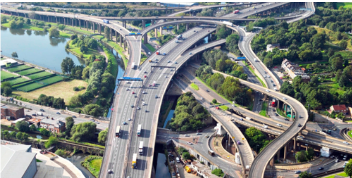
Credit: UK Highways Agency
